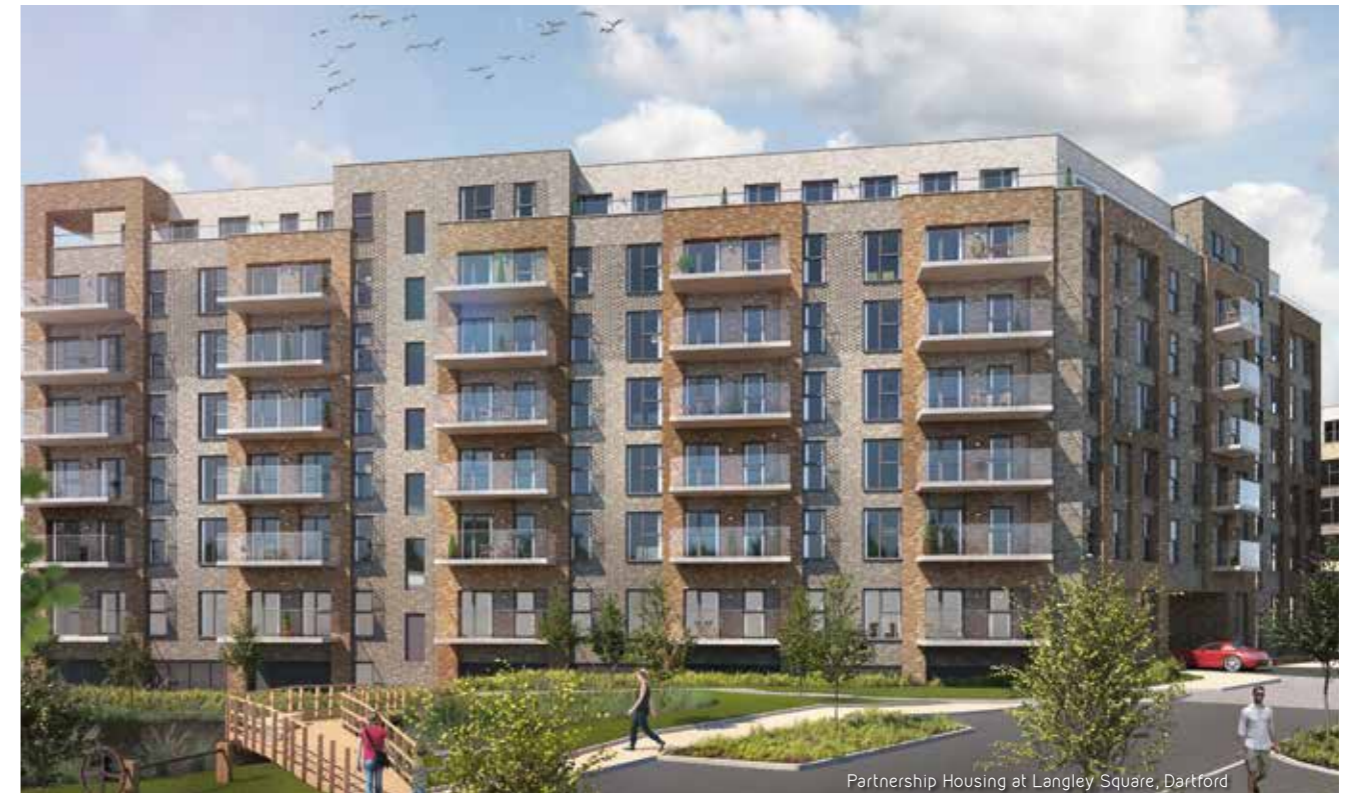
Partnership Housing at Langley Square, Dartford
