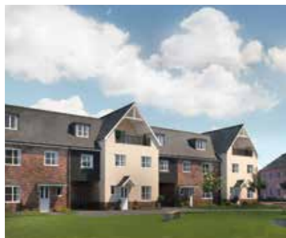
Lovats Chase, Buntingford A greenfield site close to the High Street, where we have secured permission for 56 houses and flats. There will be a new open space, retained trees, and a link to the local footpath network to cut down car use.
